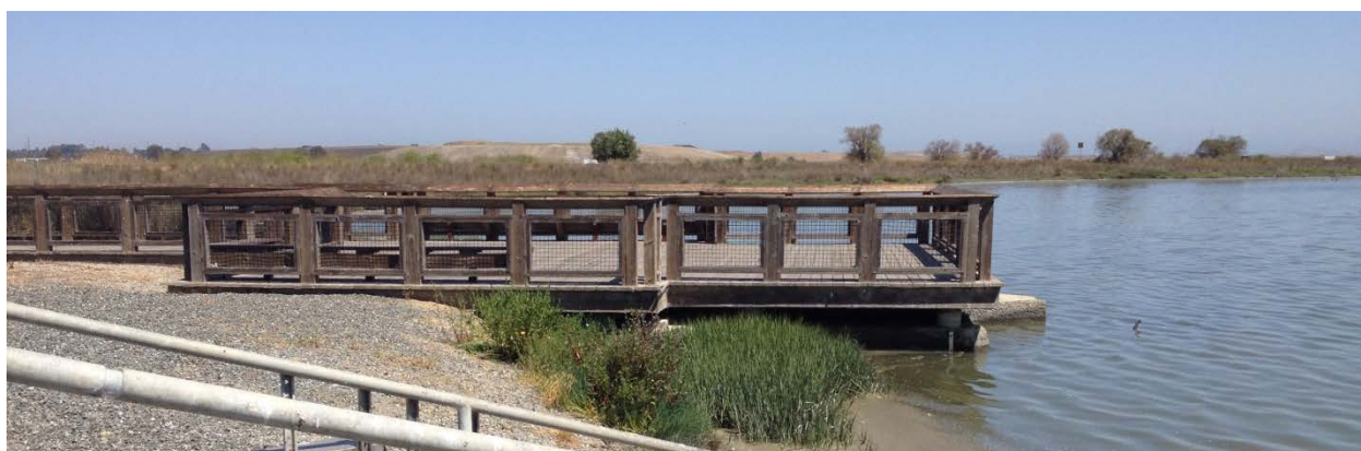
Figure 7. Photo of the Public Viewing Platform
