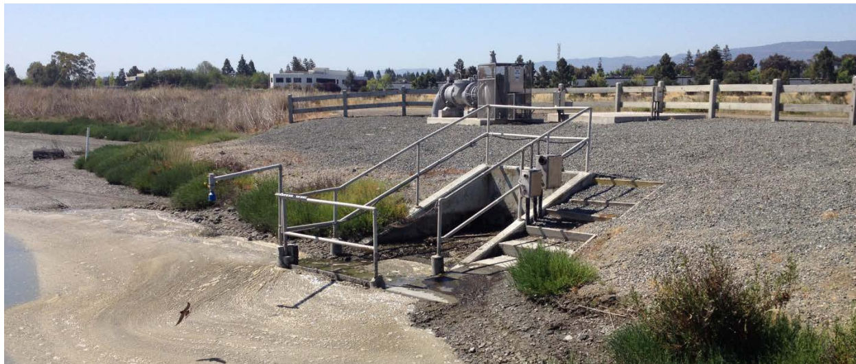
Figure 6. Photo of the Sailing Lake Pump Station’s Water Intake
