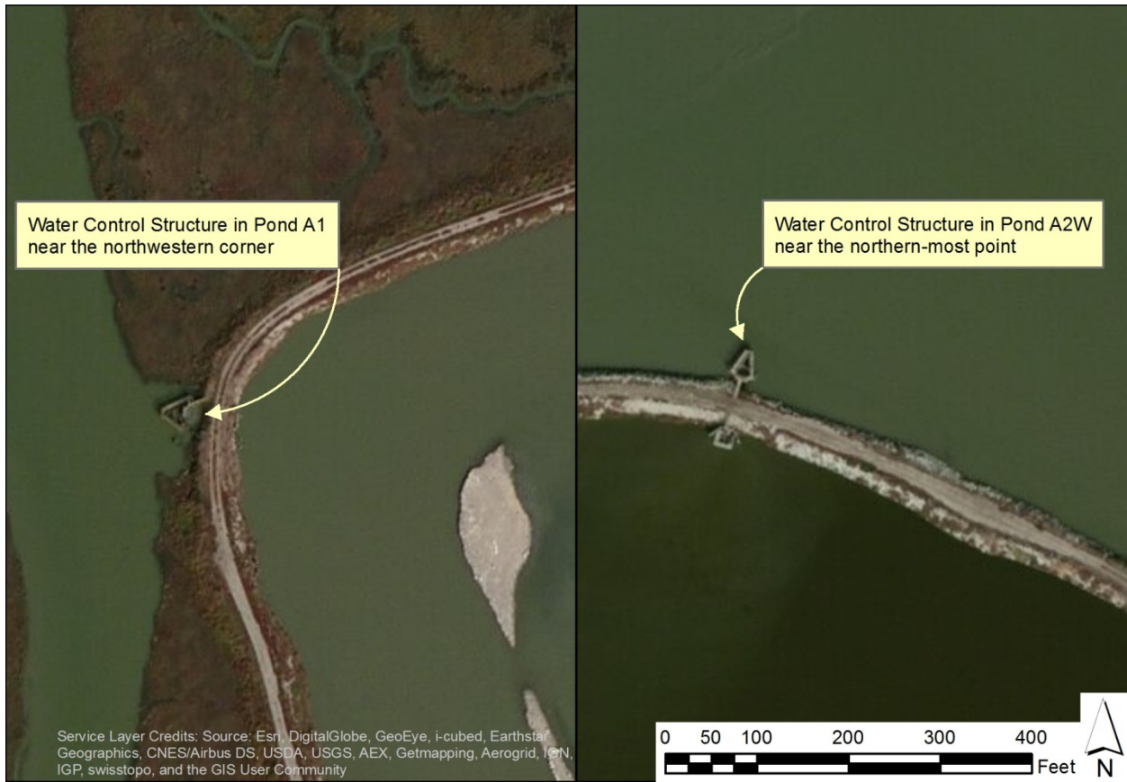
Figure 4.1. Aerial View of Water Control Structures
